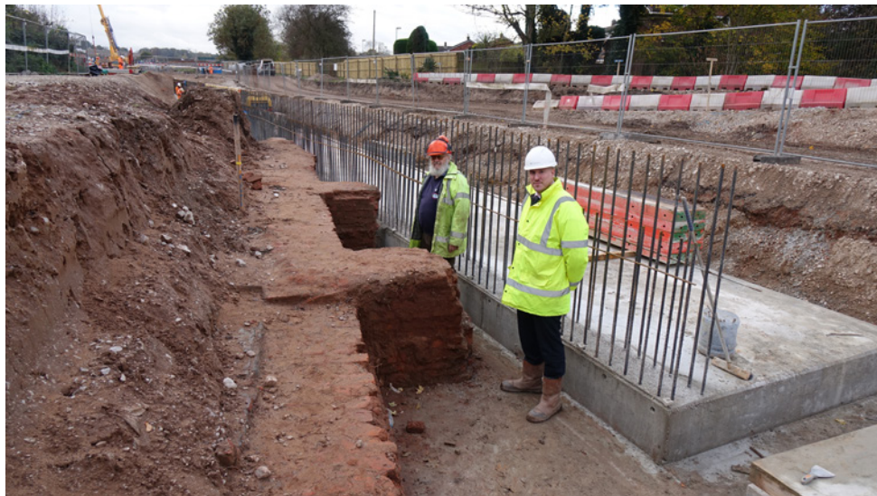
Dan Hassall, head of technical at Persimmon Homes West Midlands (right), and Peter Buck, LHCRT engineering director, stand between the newly excavated Heritage Lock 23 and the concrete base for a retaining wall which will separate the Lichfield Southern Bypass from the Lichfield Canal
